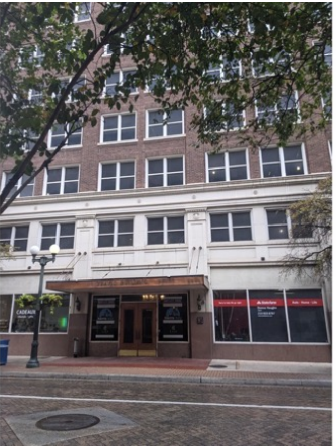
Travis Building, San Antonio $5 million
